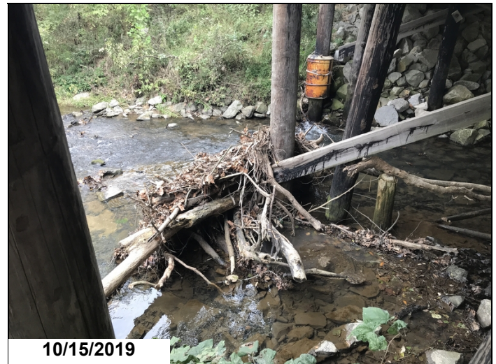
Bent 3 drift LT SIDE 2019
